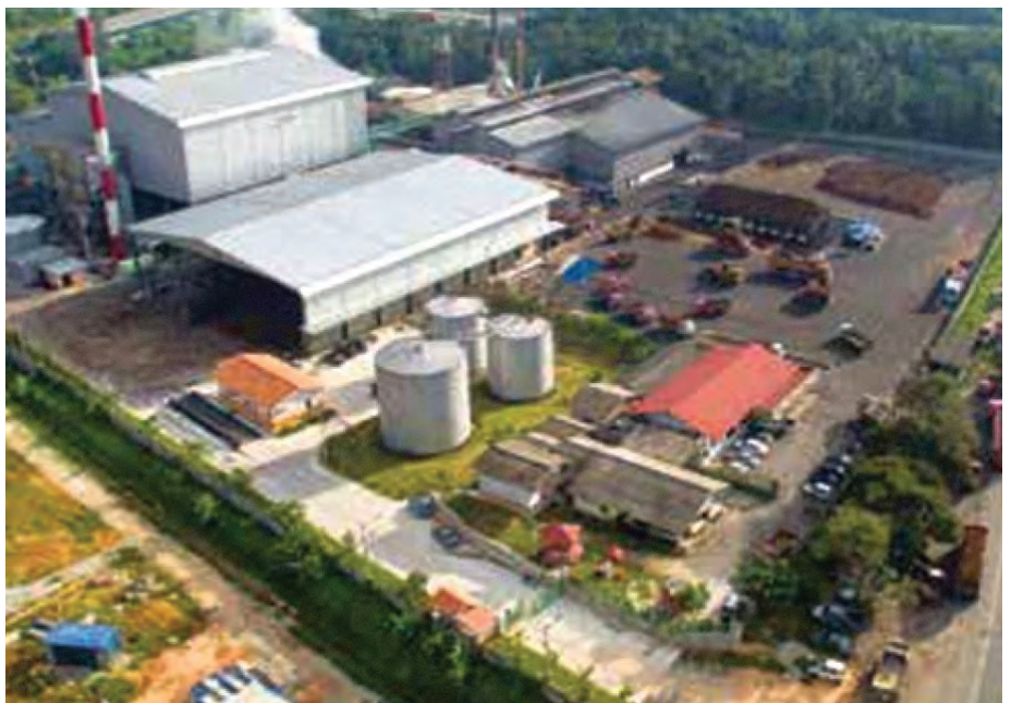
A 7MW biomass plant at Tenaga Sulpom Sdn Bhd, Dengkil, Selangor.
