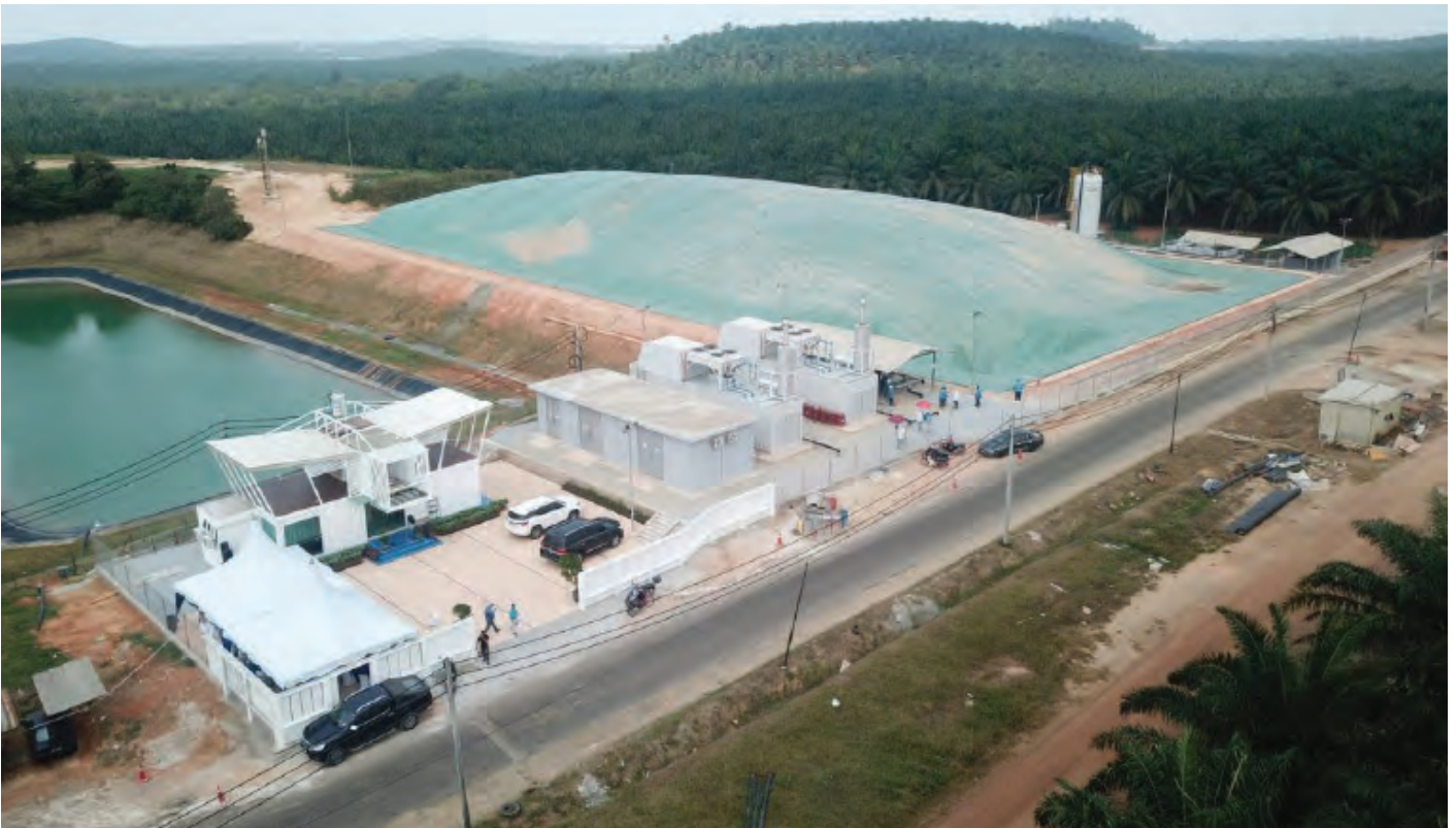
Adela Biogas Plant.
