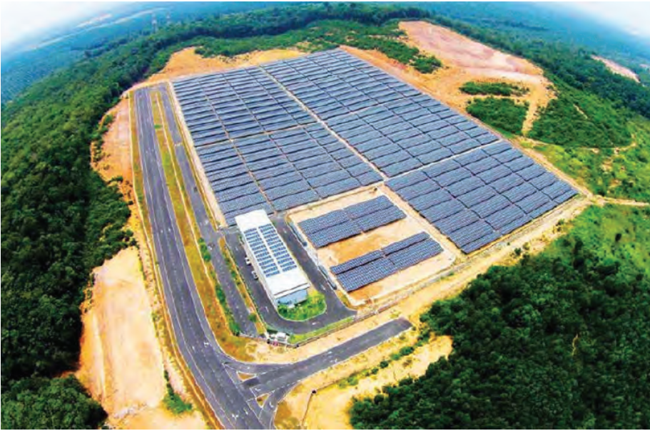
Gading Kencana 8MW Solar Farm, sprawling 17.17 acres in Melaka. (expected IOD August 2022)
