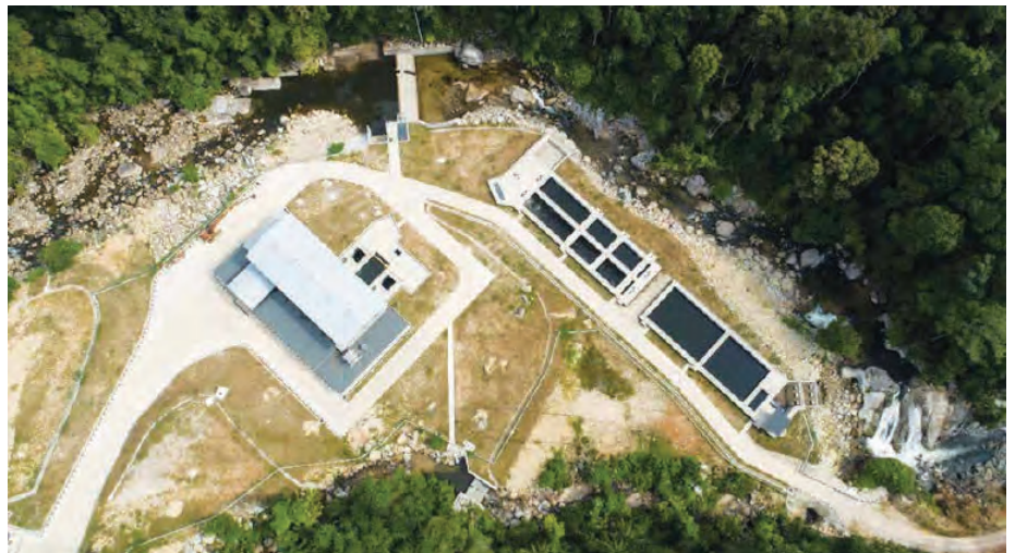
Amcorp Liang 20MW Mini-Hydro Power Plant, Raub, Pahang.
