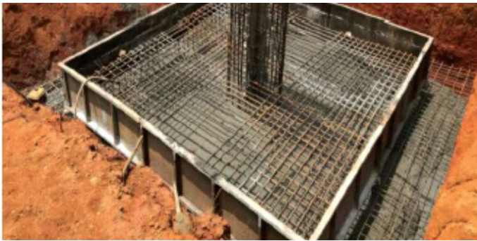
500kV OHL Ayer Tawar-Bentong South
