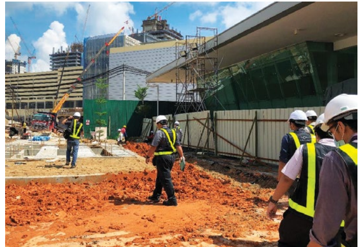
Pemasangan Tangki LPG di bawah tanah. Underground LPG Tank Installation.
