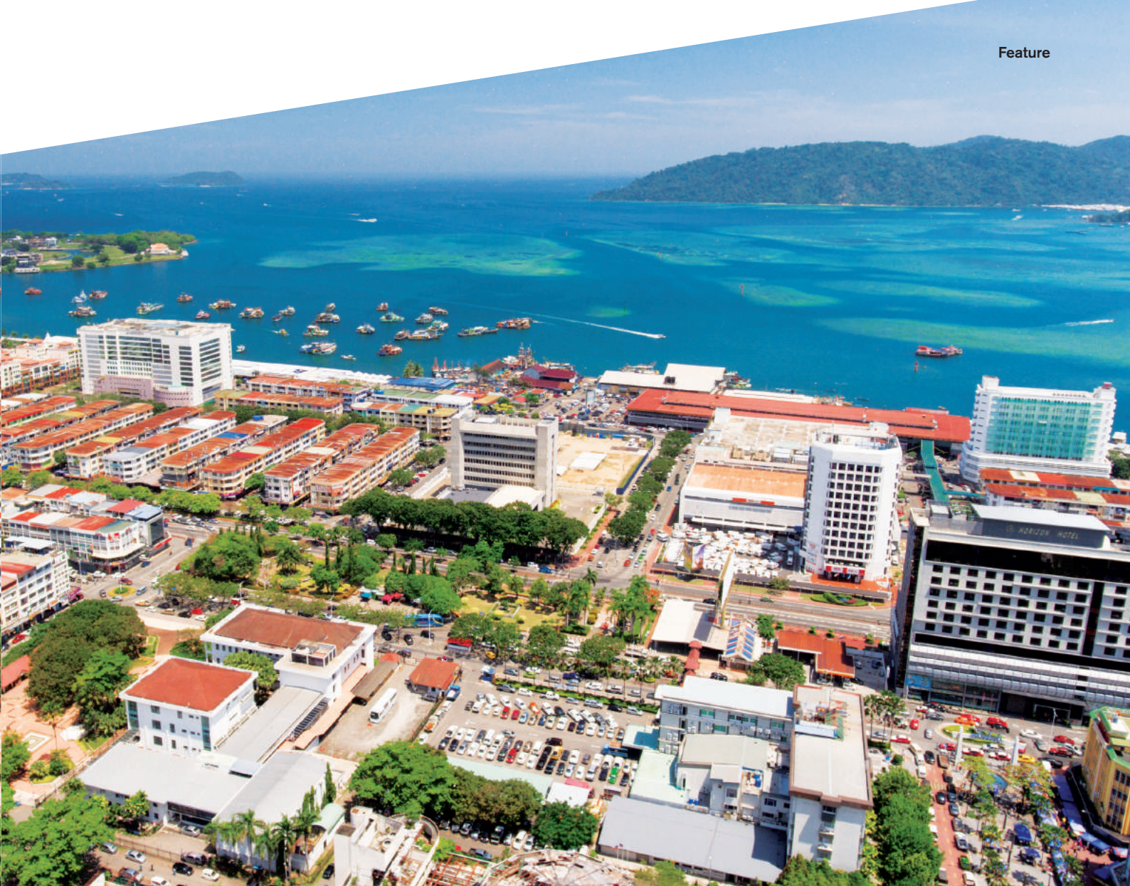
The Sabah Electricity Supply Industry has been facing various challenges and ST alongside SESB are determined to improve the SAIDI in Sabah through the SAIDI Sabah 100 Lab and TaskForce 150 (TF150).
