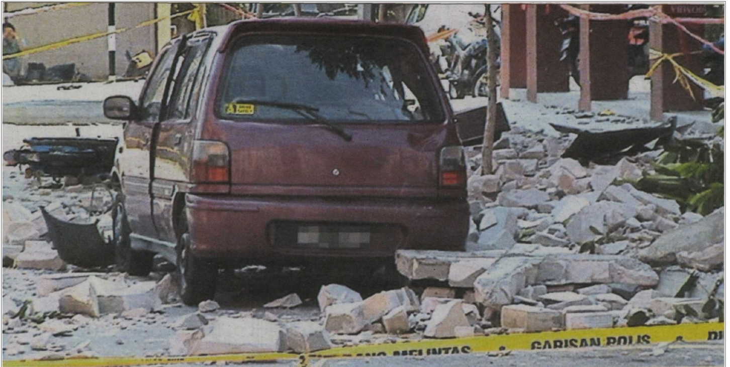
In 2004, debris fell from the roof top of a Desa Mentari apartment block after it was struck by lightning. Luckily, a car was the only casualty. — filepic
