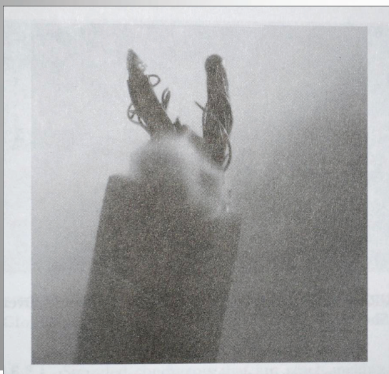
Fig (c) : Stranded Copper Conductors Severed by Arcing Through the Charred Insulation with the Strands Terminated in Beads.
