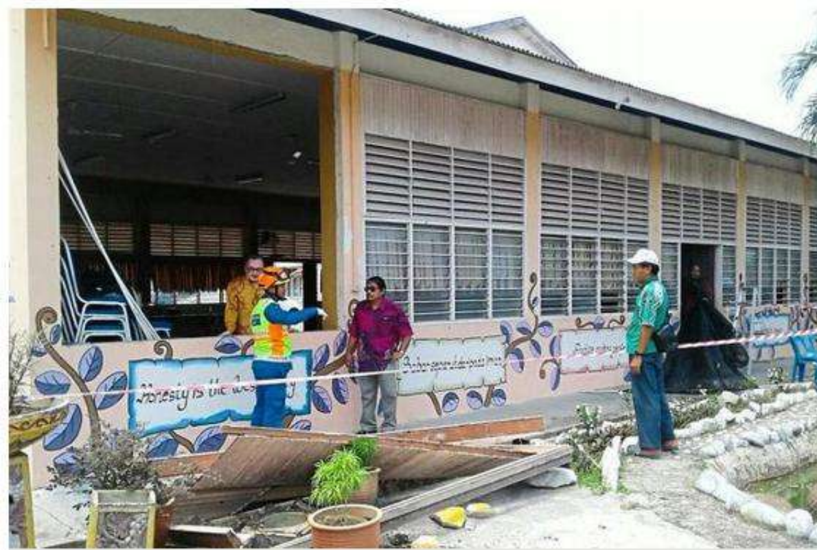
Damaged: A fireman talking to school officials at the scene.
