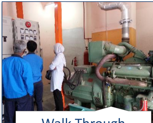
Walk Through Energy Audit
