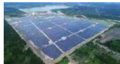
LSS Sepang - Malaysia's largest solar plant
