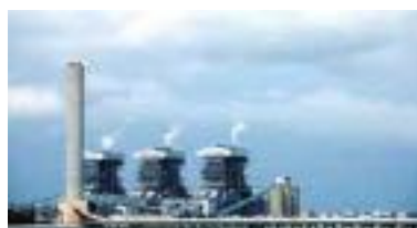
The 3,100 MW coal-fired plant SJSAS Manjung in Perak. The original installed capacity for this plant started with 3x690MW, M4 (1x1010MW) COD in 2014.
