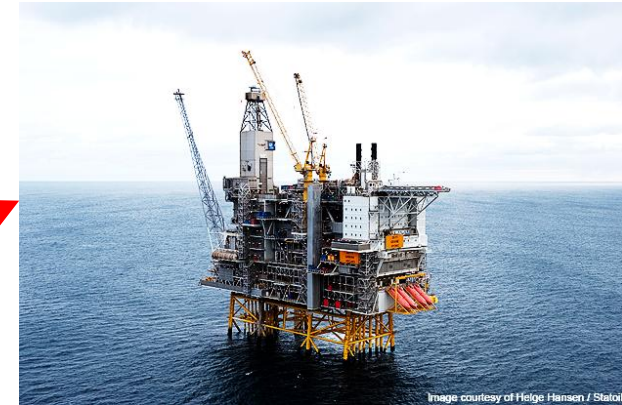
Oil & Gas Platform
