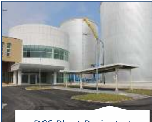
DCS Plant Project at KLIA2
