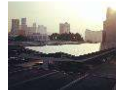
Solar PV @ Car Park, TNB Head Quarters Bangsar, Kuala Lumpur
