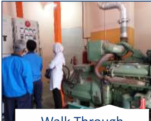
Walk Through Energy Audit
