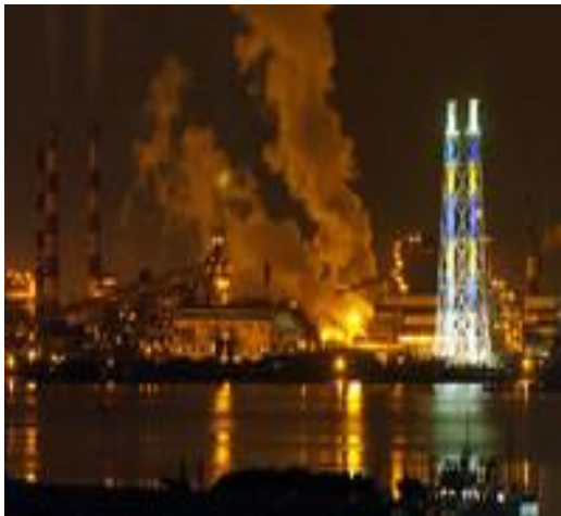
A steel factory at night in Pohang in Korea
