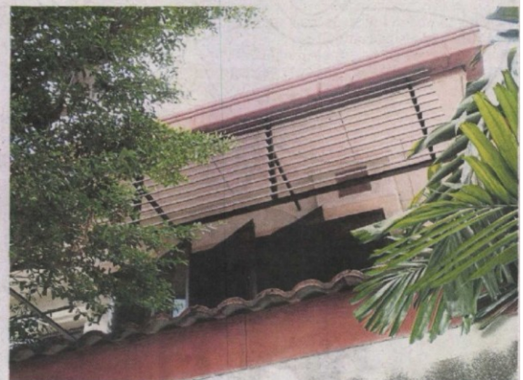
An awning or sun louvres will provide more cooling shade for your home, especially for windows that face the rising or setting sun.
